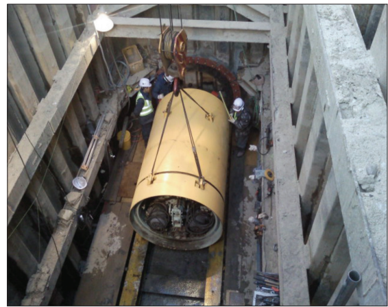
Shield Tunneling Body Setting
